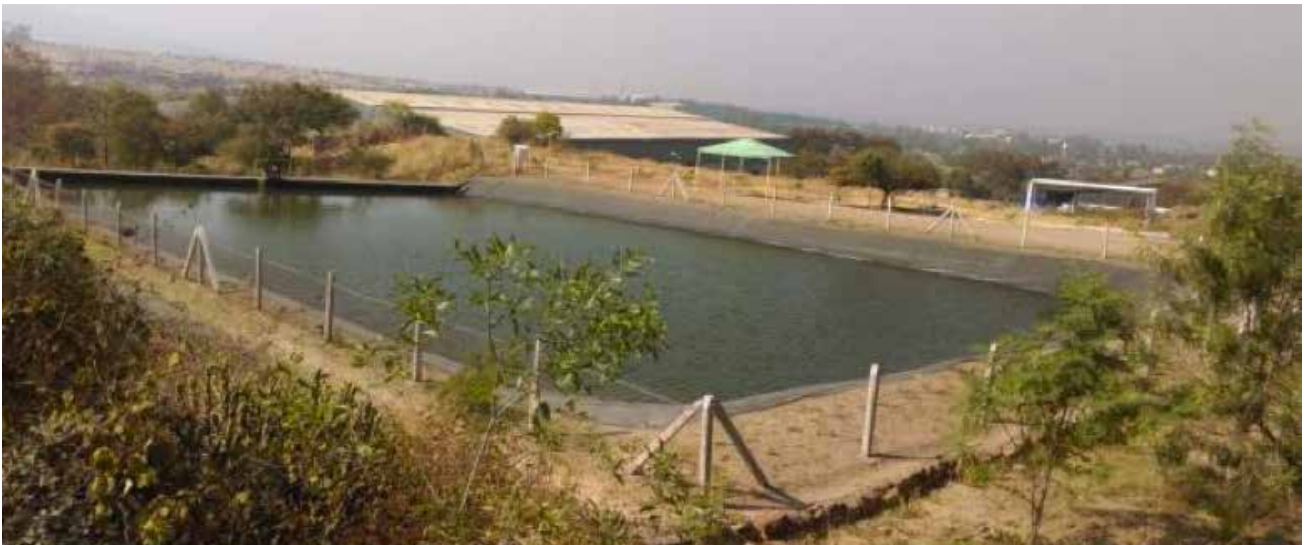
Rainwater harvesting at Shirwal
