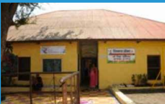
Parapet railing for additional safety
